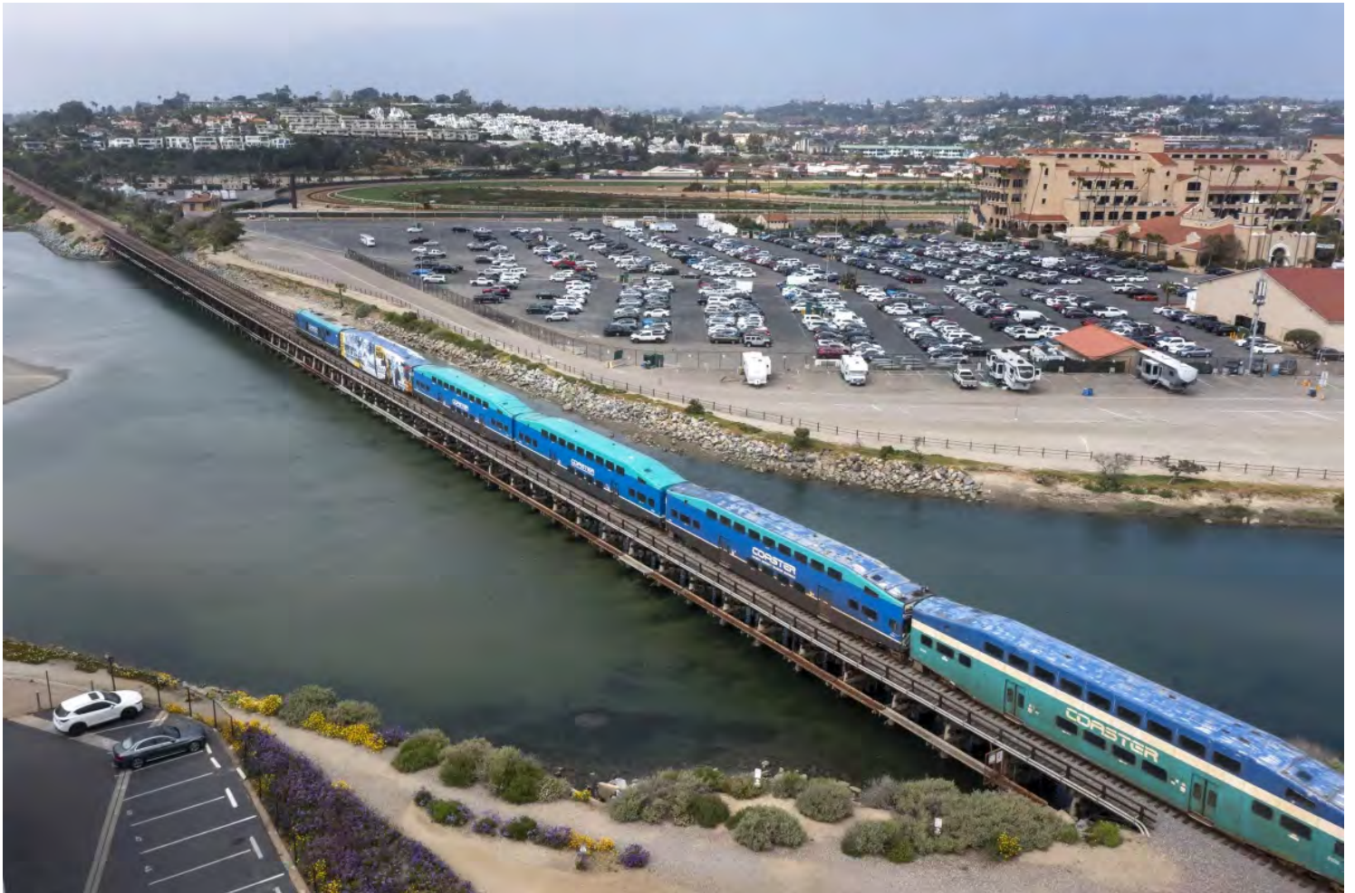
A Coaster train crosses the San Dieguito River Railway Bridge in Del Mar on Wednesday. (K.C. Alfred / The San Diego Union-Tribune)
