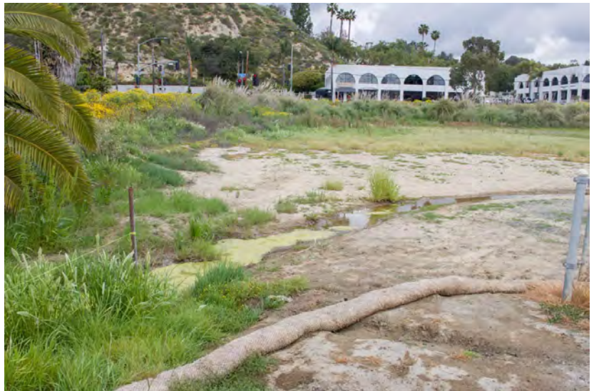
Surf Cup Sports leaders were cited for violating the Clean Water Act after redirecting stormwater into a swale that leads to the San Dieguito River. Photo by Laura Place
